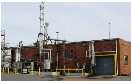
Manufacturing Facility on Chelsea Ave
