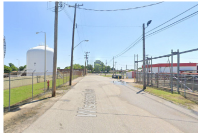
Industrial Facility on Riverside
