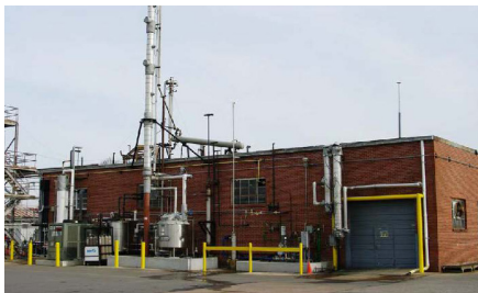
Manufacturing Facility on Chelsea Ave
