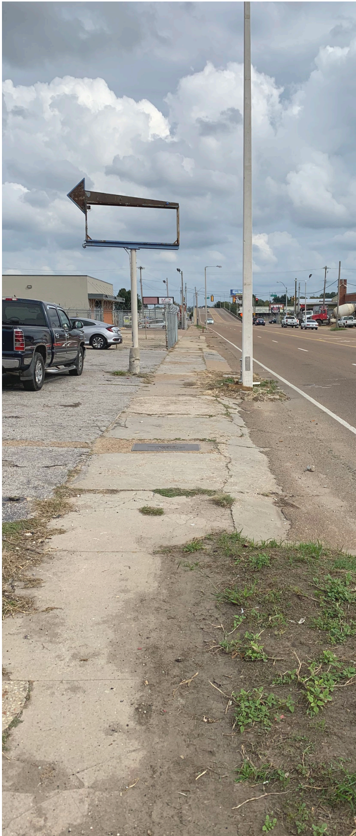
Summer Avenue today - looking east. Poor pedestrian infrastructure.
